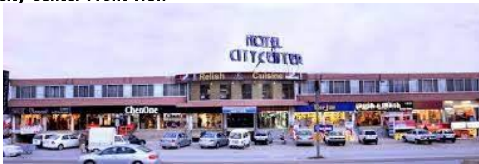
Figure 20: City Center Front view
