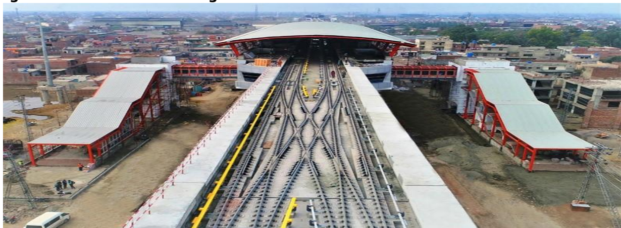
Figure 5: Tracks of the Orange Line
