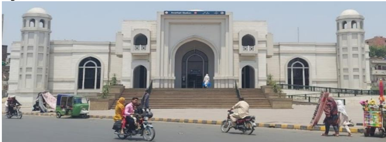
Figure 6: View of Anarkali Station
