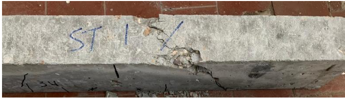
Figure 6: flexural cracks that occurred on Steel beam (1)
