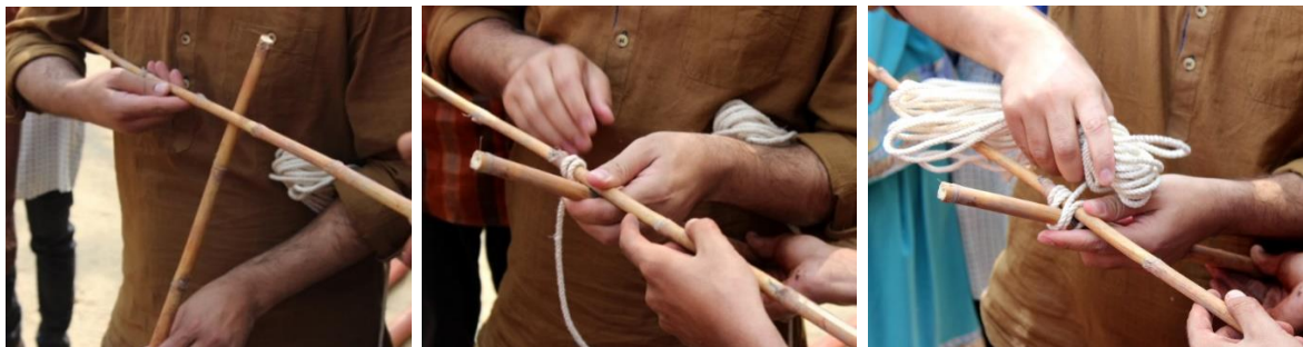
Figure 15 (a)(b)(c): Important Technique of Joining Bamboos through Different Knots and Lashing with Ropes Source: (Author)
