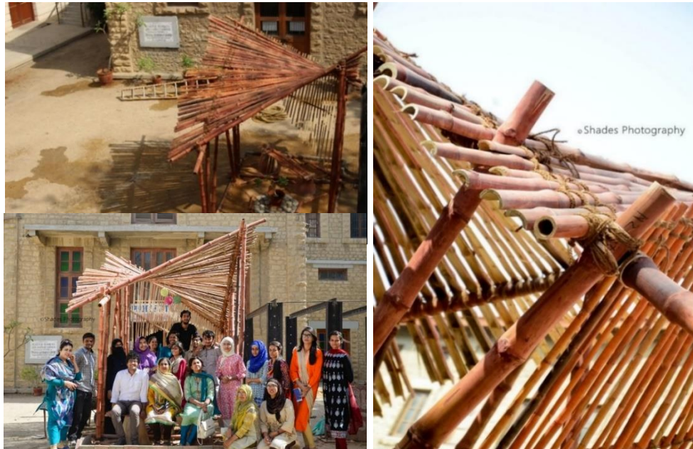
Figure 19 (a)(b)(c): Students Pavilion has been Erected, Highlighting the Bamboo Structure, its Joineries, Lashing, Landscape Features, Benches and Final Group Photo Along with the Author/Instructor of the Project
