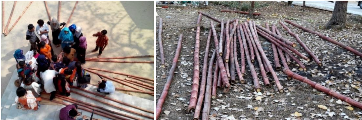
Figure 9 (a) (b): Bamboo Poles on Site and Student Discussion to Devise Strategy for Cutting on Measurement
