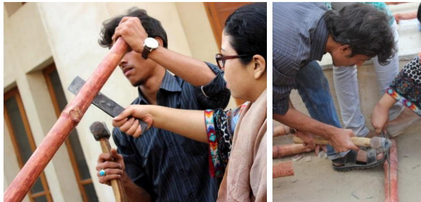
Figure 13 (a) (b): Basic Technique of Split Bamboo
