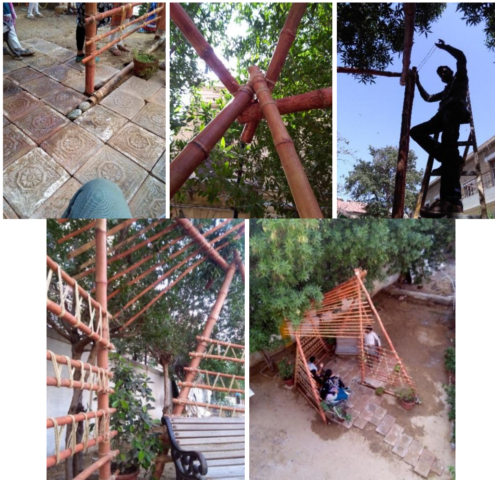
Figure 18 (a)(b)(c)(d)(e): Students Pavilion has been Erected under the Tree Shade, Highlighting the Bamboo Joineries, Lashing and the Clay Tiles used for Flooring
