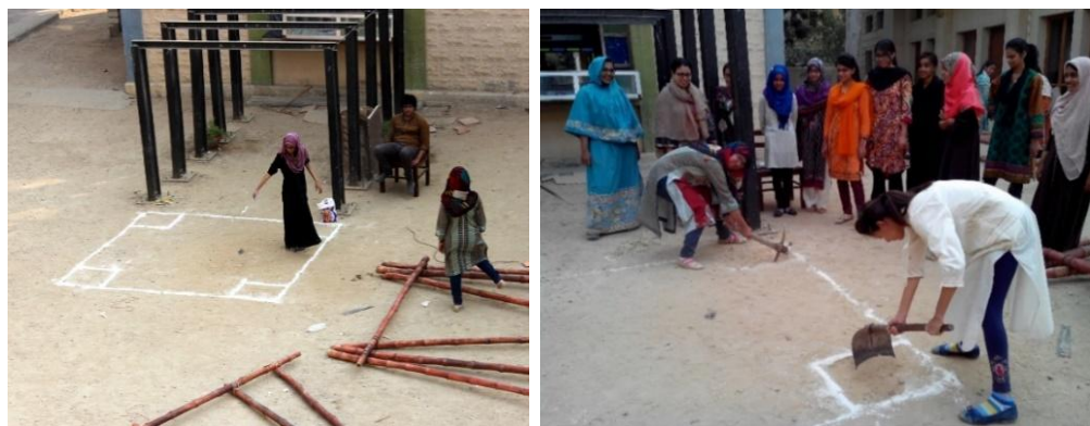
Figure 16 (a)(b): Site Layouts and Excavation for Bamboo Posts Foundation Source: (Author)
